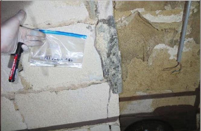
1. OG, Innenwand, Putz (Probe P 23: Asbest n.n.)
