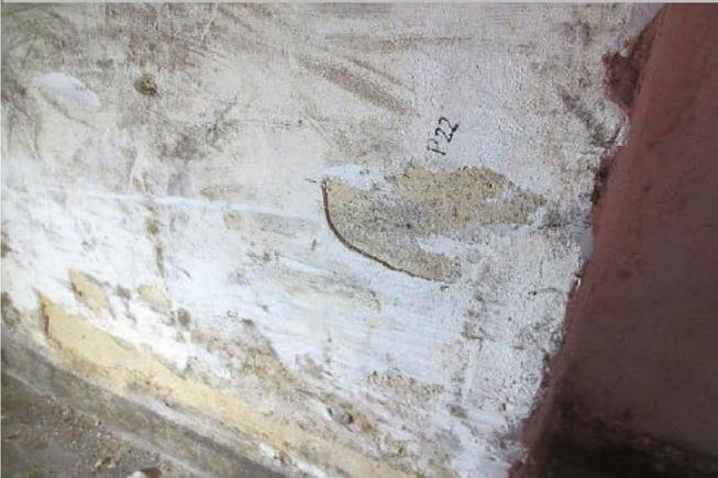
1. OG, Innenwand, Putz (Probe P 22: Asbest n.n.)
