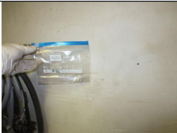
Nr. 140, Anbau: Souterrain, Wandputz → P 06
